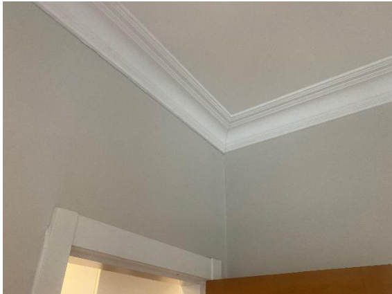
Figure 21: Later but sympathetic cornice on wall to be removed (Source: Three + One Heritage, 26.08.24)
